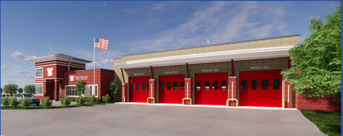
New Fire Station
