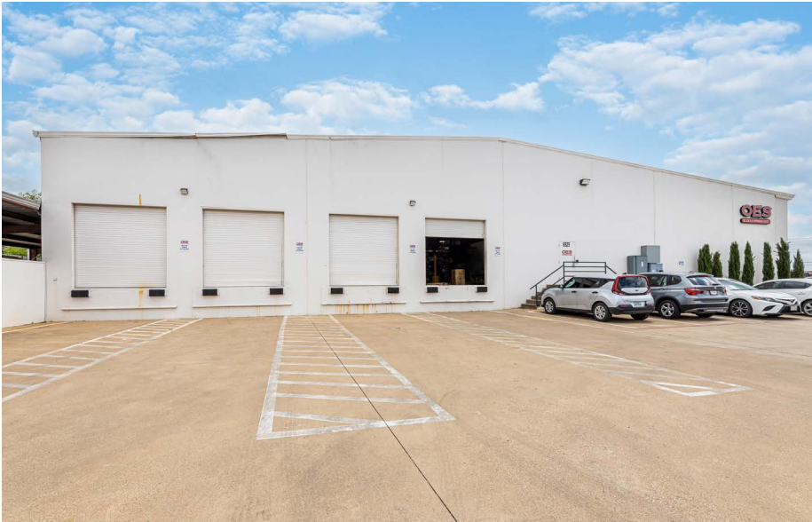
West Side Truck Court - Dock High
