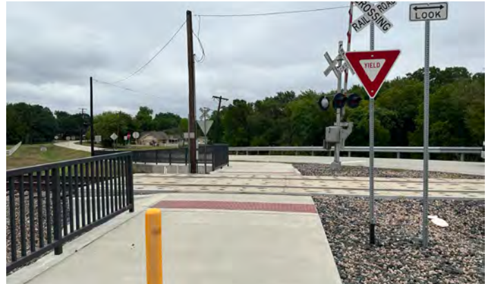
Pedestrian crossing on rail in Murphy, Texas
