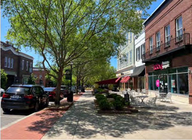
Urban sidewalk example in Baxter Village, South Carolina
