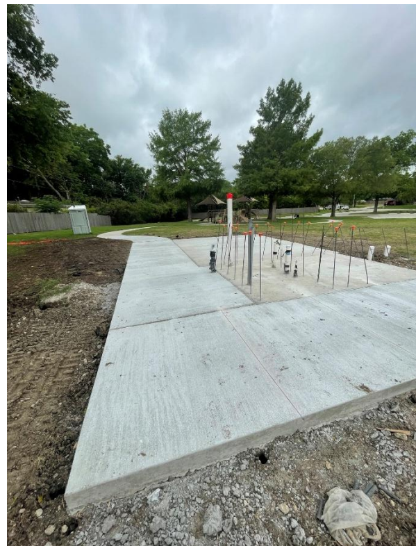
Kate Baker Park Restroom Foundation
